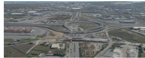
K16 junction of PATHE highway and the inner Thessaloniki ringroad
