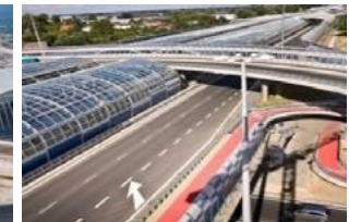
Construction of the road S8 – the ARMII KRAJOWEJ Route, Poland
